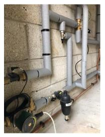
New primary pipework was installed and connected to the existing 15mm copper system throughout the house. All radiators were resized and replaced. As the ASHP is circulating water at a lower temperature the radiator sizes were increased by c.100%. The whole system was flushed and cleaned with a special cleaner before commissioning.
